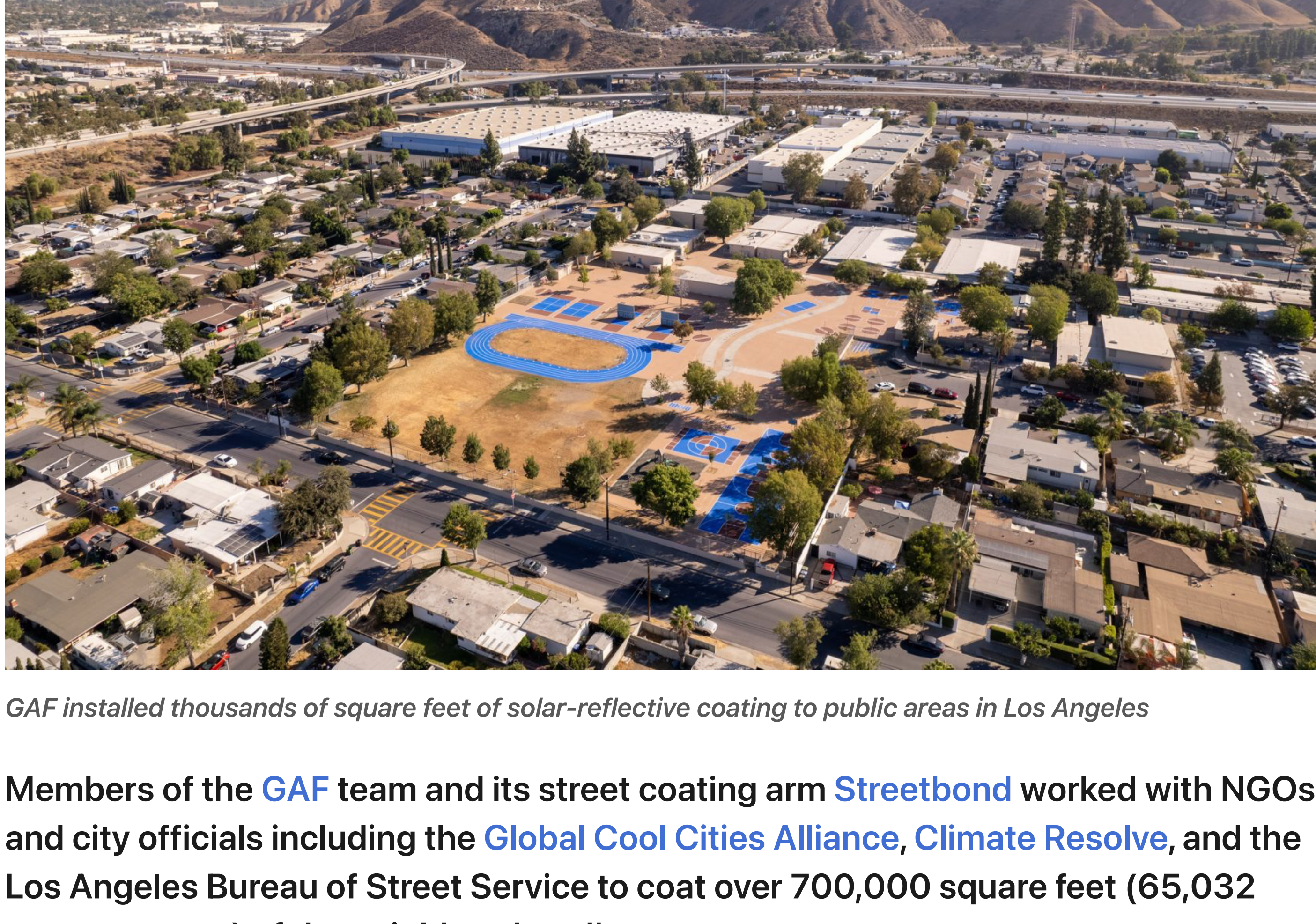
GAF installed thousands of square feet of solar-reflective coating to public areas in Los Angeles
