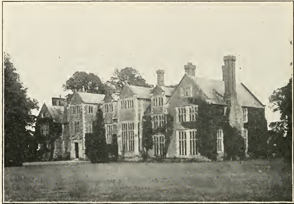
LOSELEY PARK, NORTH FRONT
