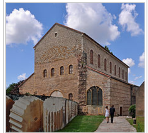
Basilica of Saint-Pierre-aux-Nonnains in Metz, where Louis the Pious was buried.
